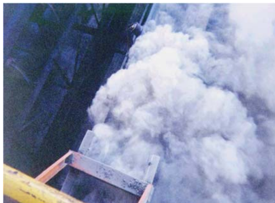
Figure 3. Dust plume due to improper transfer design
