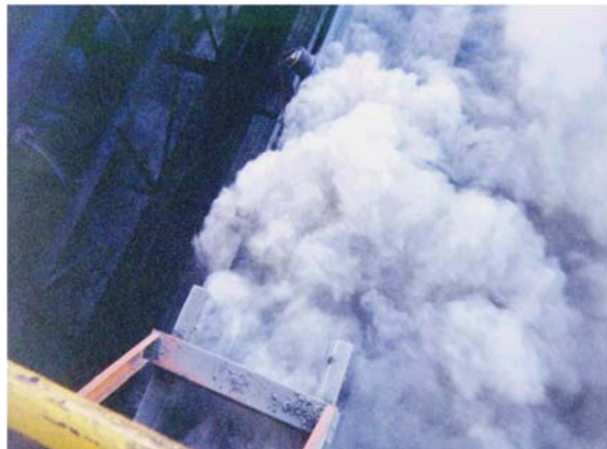
Figure 3. Dust plume due to improper transfer design
