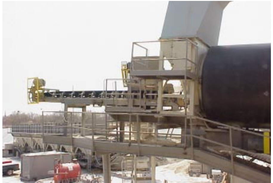
Asphalt plant slinger presents tough, demanding application for conveyor belt cleaners.
